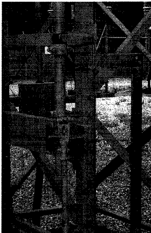
Figure 36—Typical brailess grounding device
